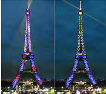
Figure 11.2-1 The Eiffel Tower of Paris, locally known as la dame de fer , illuminated by LED lighting. This 330-m high tower, erected as the entrance arch for the 1889 World's Fair in Paris, may well be the most recognizable structure in the world. Over the years, the iconic shape of the Eiffel Tower has successively been highlighted by gas lamps, incandescent lamps, fluorescent lights, high-pressure sodium-vapor lamps, and now by a programmable, dynamic LED lighting system that is synchronizable with music and sound.
